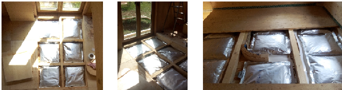
Fig. 4: Macroencapsulated PCM integrated in the floor compartments (left, middle) and in the intermediate ceiling (right).
