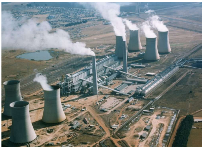
Figure 3: Hendrina Power Station (Eskom, 2025)
