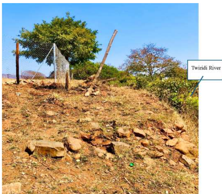
Fig. 1: Fence that has moved due to heavy floods. Source: Author, 2025
