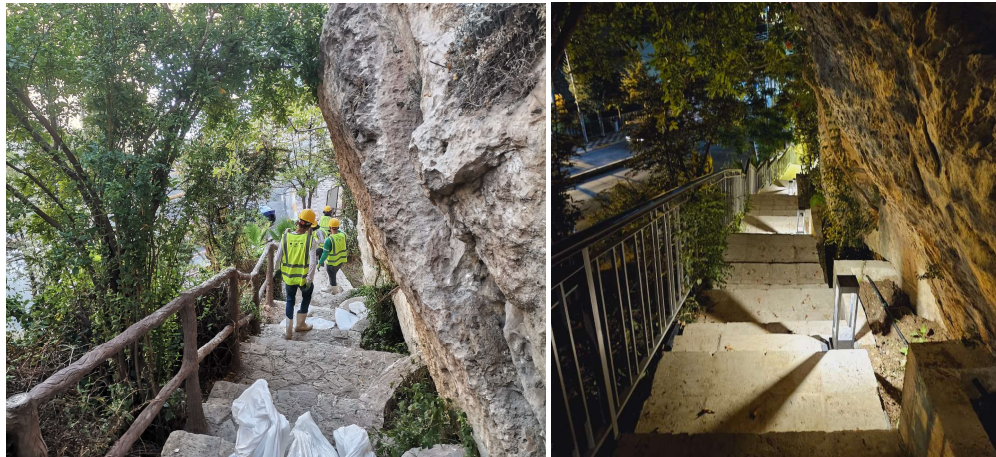
Fig. 7: Stone stairs. The before and after intervention.
